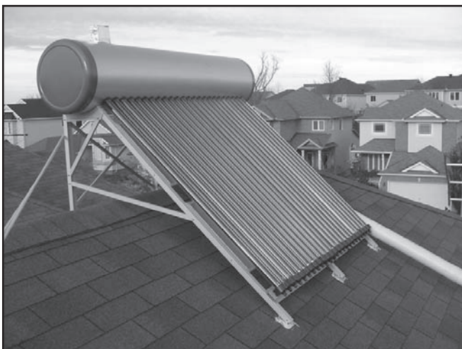
Figure 10. The Globe Solar Energy IP-195 can be ground mounted or placed on a rooftop, as pictured here. The user-supplied insulated and heated unibical can be seen leading from the unit at lower right.
