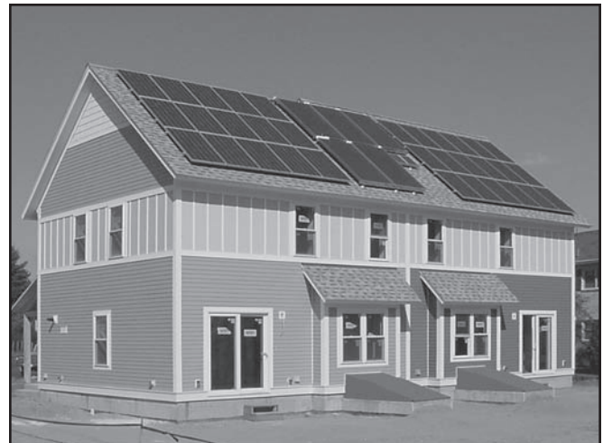
Figure 1. The 20 duplex units at Wisdom Way Solar Village are designed for low- and moderate-income buyers. Except for a box bay on the side of each unit, the shape is a simple rectangle, making for efficient framing and air sealing.
